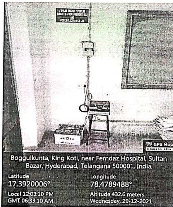
Inverter and AC&DC Box of solar plant
