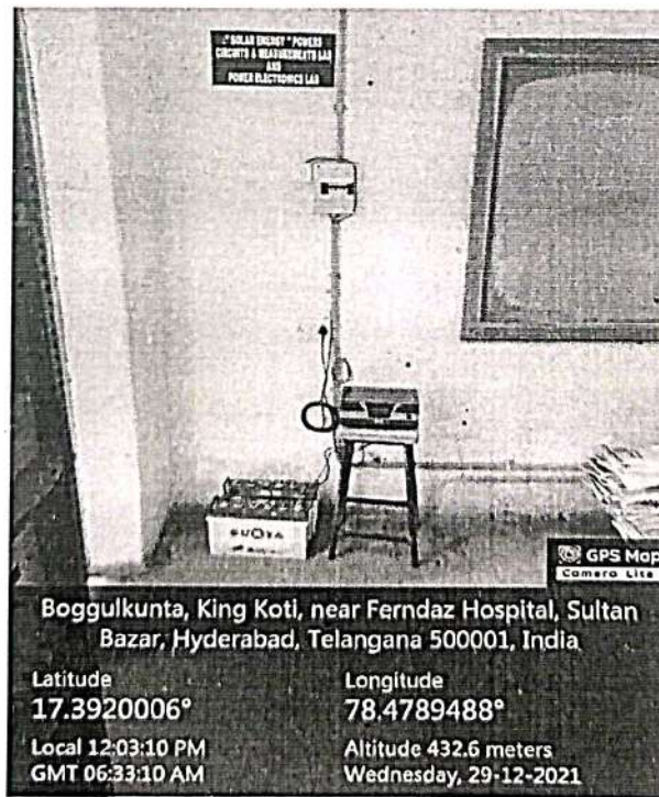
Inverter and AC&DC Box of solar plant
